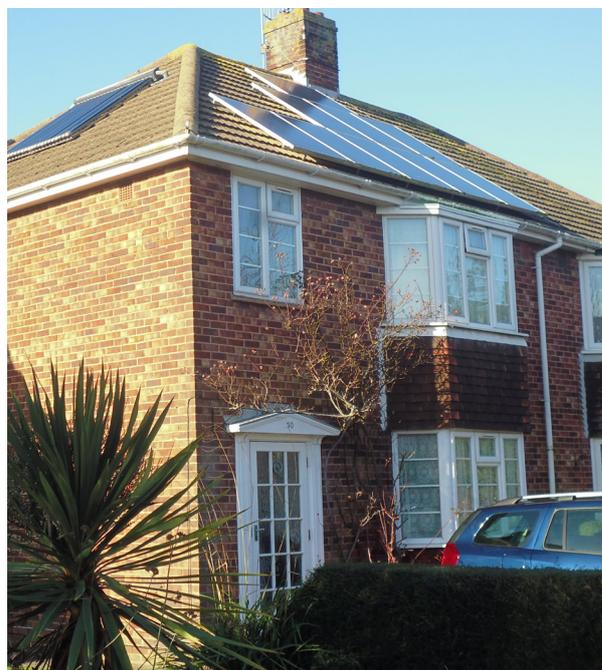
The PV panels generate around 3200kWh per annum which, together with their solar thermal providing much of their hot water and the insulation measures, give them a very low carbon lifestyle which was their primary motivation, but they have gained so much more along the way.
